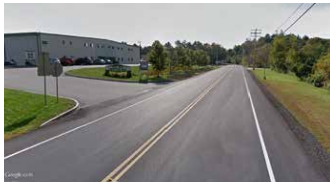
Heritage Ave is a typical example of this roadway typology in Portsmouth.
