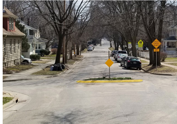
An alternative to the raised intersections includes installation of mini-roundabouts intended to slow traffic as it passes thru low-volume intersections (photo from Madison WI)
