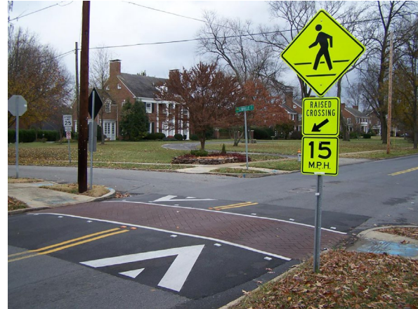
Example photo of a raised crosswalk that is recommended for installation at the south leg of the McKinley/Harding intersection
