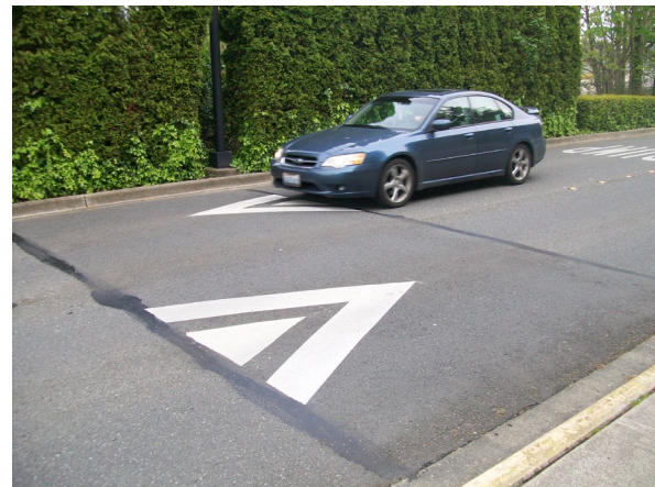
Strategically-placed speed humps are recommended along McKinley Road to slow traffic speeds
