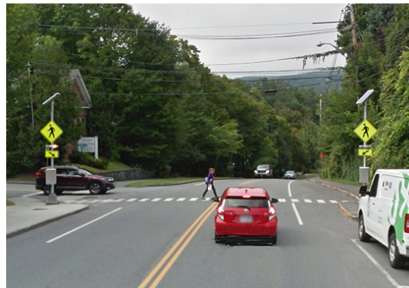
Example of a crosswalk with Rectangular Rapid Flashing Beacons (RRFB) in Hanover NH (Google Streetview image)
