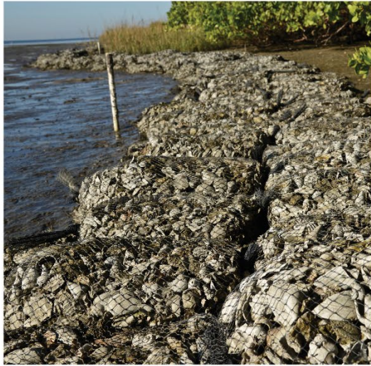
GABIONS WITH OYSTER SHELL AND ROCK
