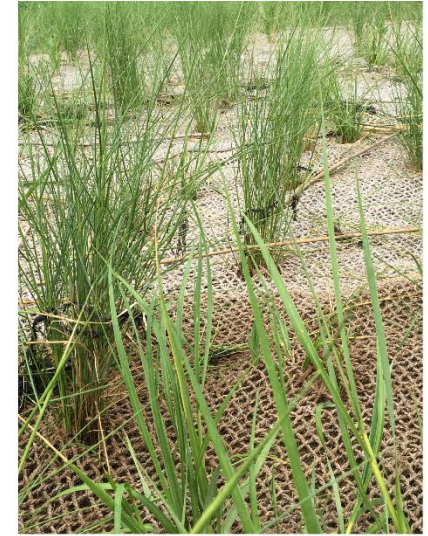
MARSH GRASS PLANTINGS INSTALLED WITH COIR BLANKET
