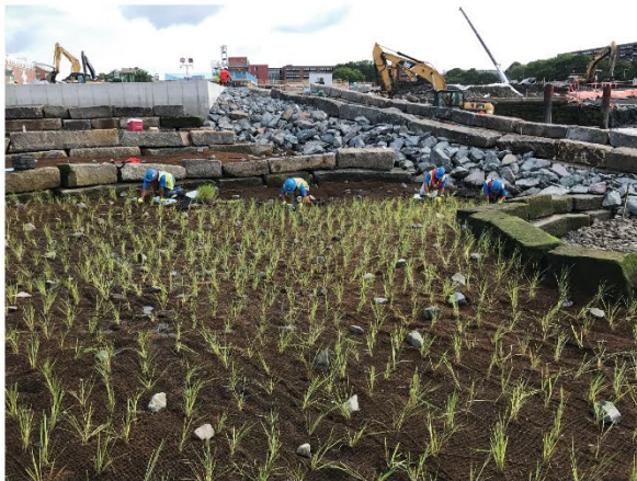
SALVAGED GRANITE BLOCK CELLS
