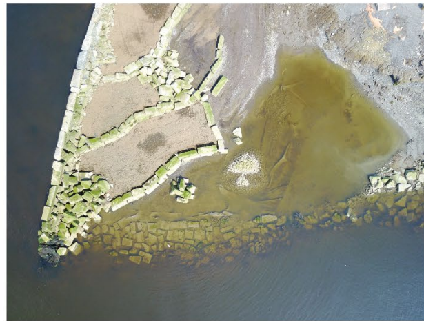
SALVAGED GRANITE PLANTING BEDS ESTABLISHED WITH PLANTING MEDIUM INSTALLED
