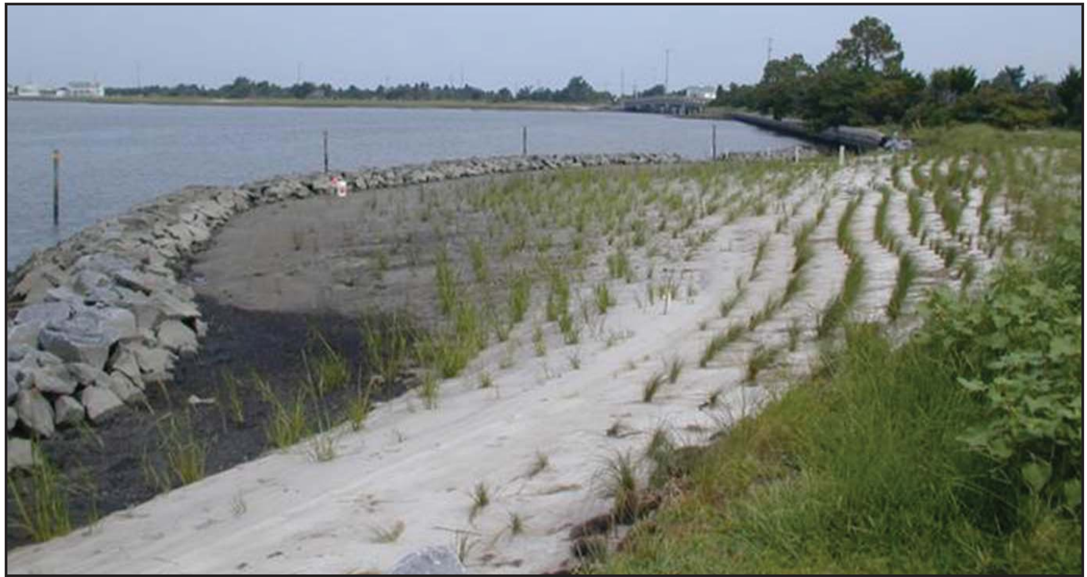
BOULDERS AS SILL STRUCTURE | PROPOSAL WILL BE TO USE WIRE GABIONS FILLED WITH OYSTER SHELL
