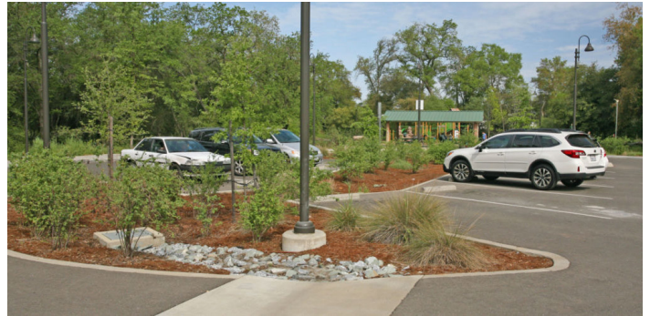
Above: A simple curb cut allows plants to filter stormwater that enters this open space's parking lot; Arcade Creek Preserve, CA.
