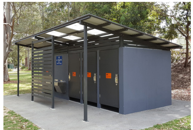
Above: An example of solar powered restrooms with roof mounted solar panels.
