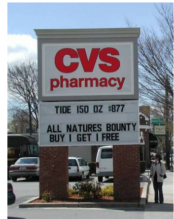
Total width of supports is greater than 1/3 of the width of the sign – Included in sign area
