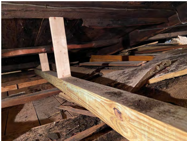
13 – New 4x4 and purlin shoring
