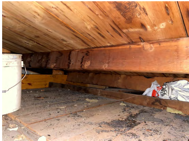
14- View of repaired roof framing
