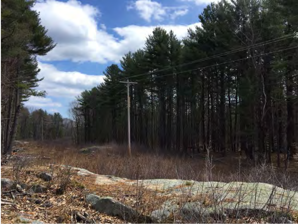
Photo 26. Facing east down transmission right-of way (4/15/2020)
