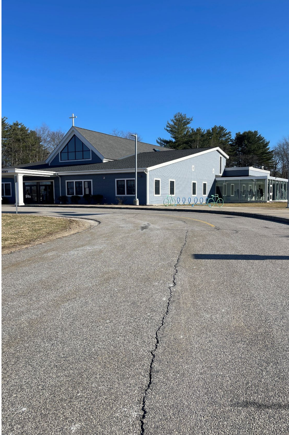
Front Elevation of School Building (Showing area of proposed addition)
