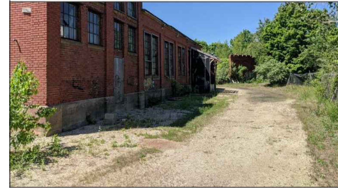
Photograph No.: 13 Date: 6/17/20 Direction Taken: South
