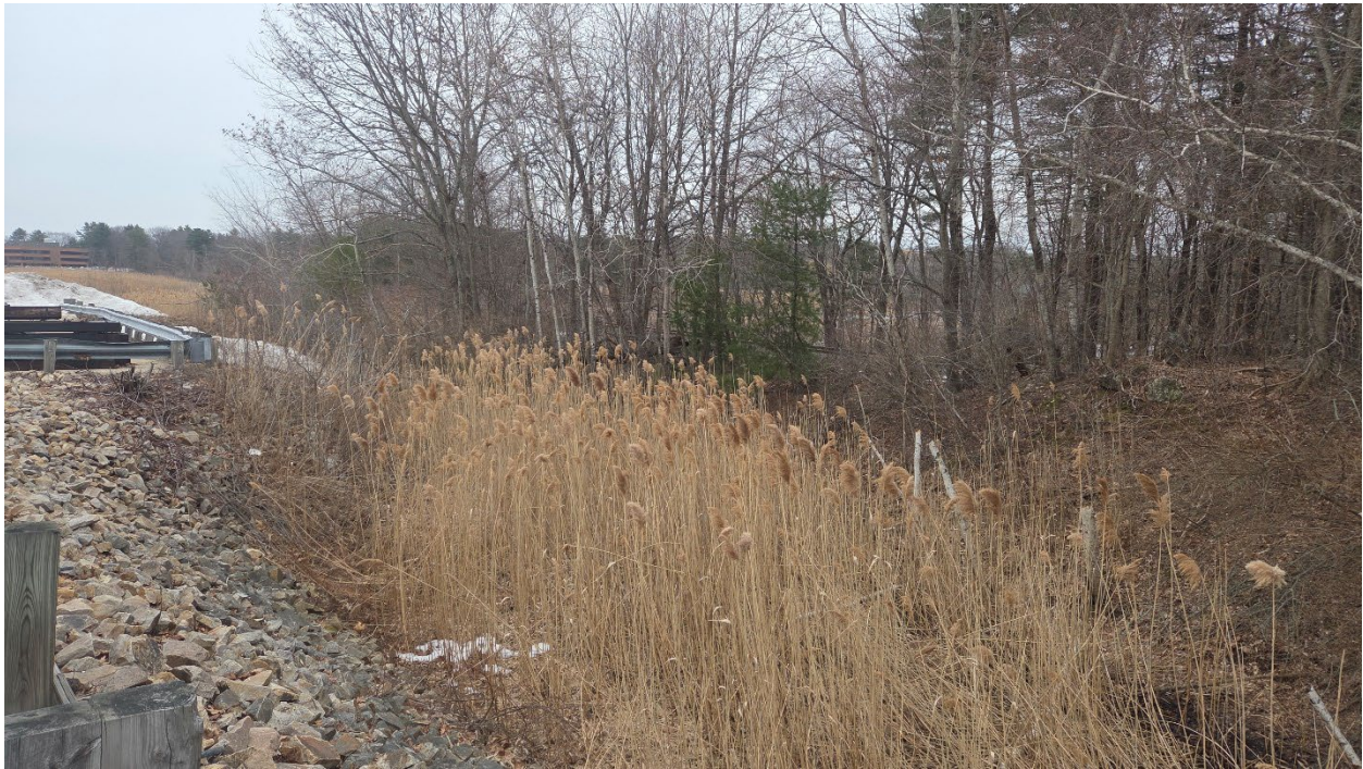
Photo 5 – Liberty Mutual – View looking east along the Stormwater Area (Photo taken 3/20/2026).
