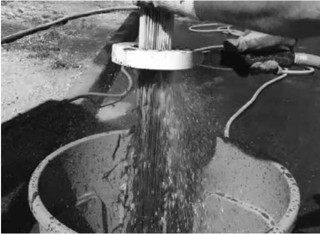
Rinsing Cartridge with Contech Rinse Tool
