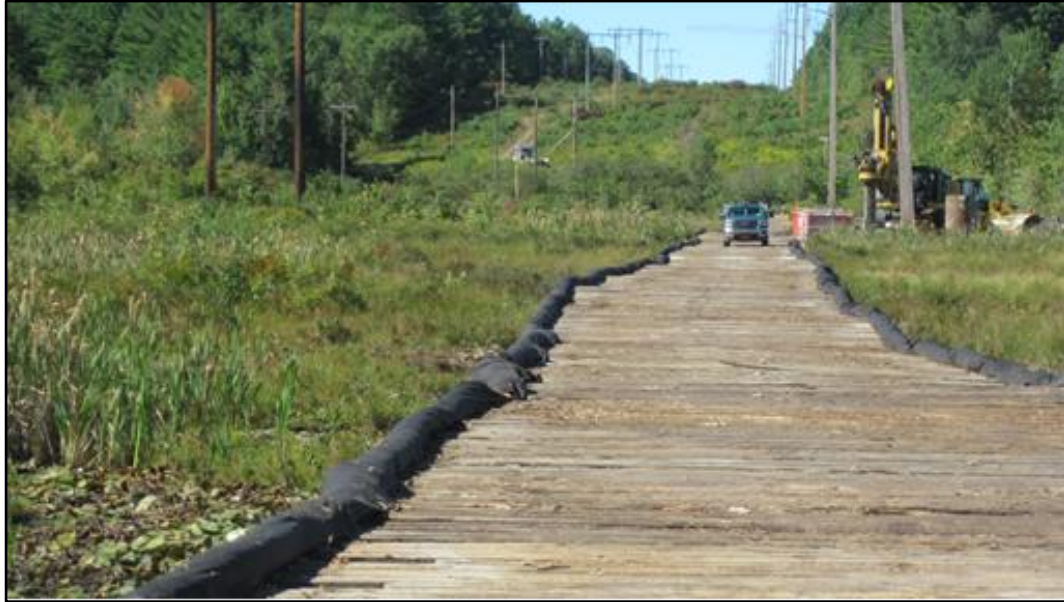
Swamp mats with coir logs wrapped in filter fabric to create a temporary curb. Turtle Town Pond, Concord, NH. Credit: Karl Benedict
