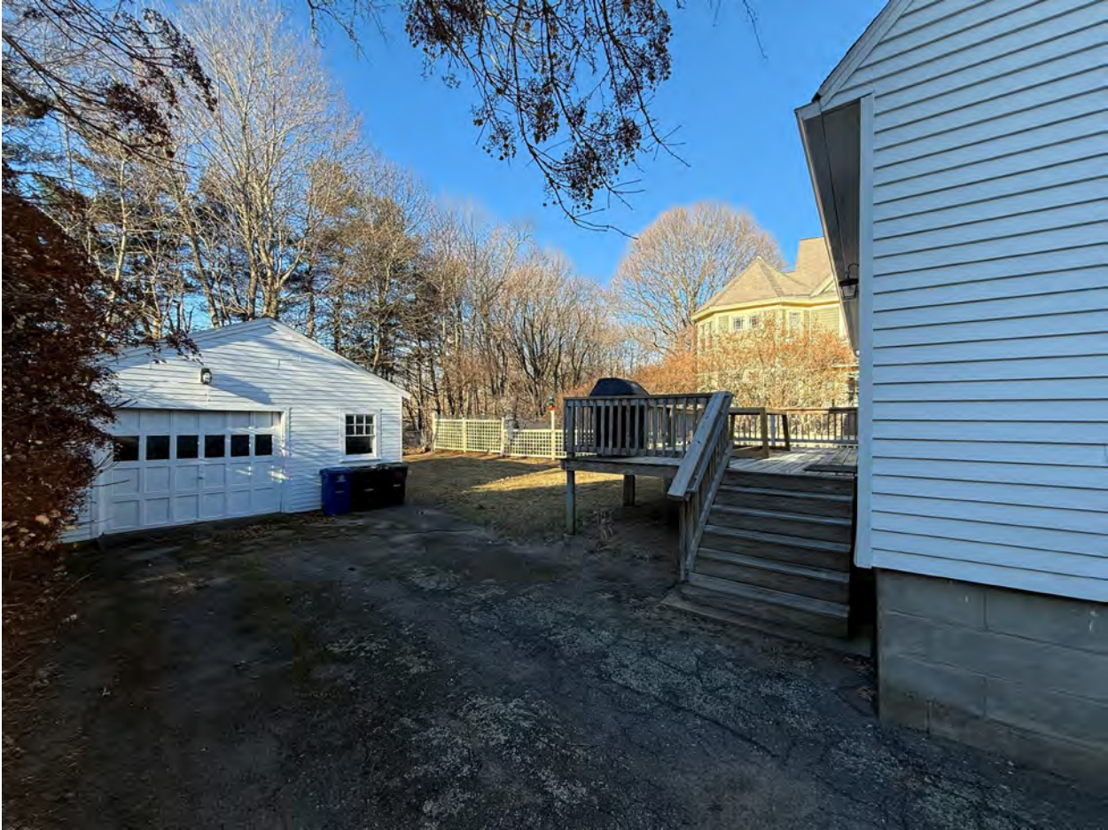
Existing Garage & Rear Deck
