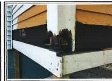
Deteriorated Wood on Porch
