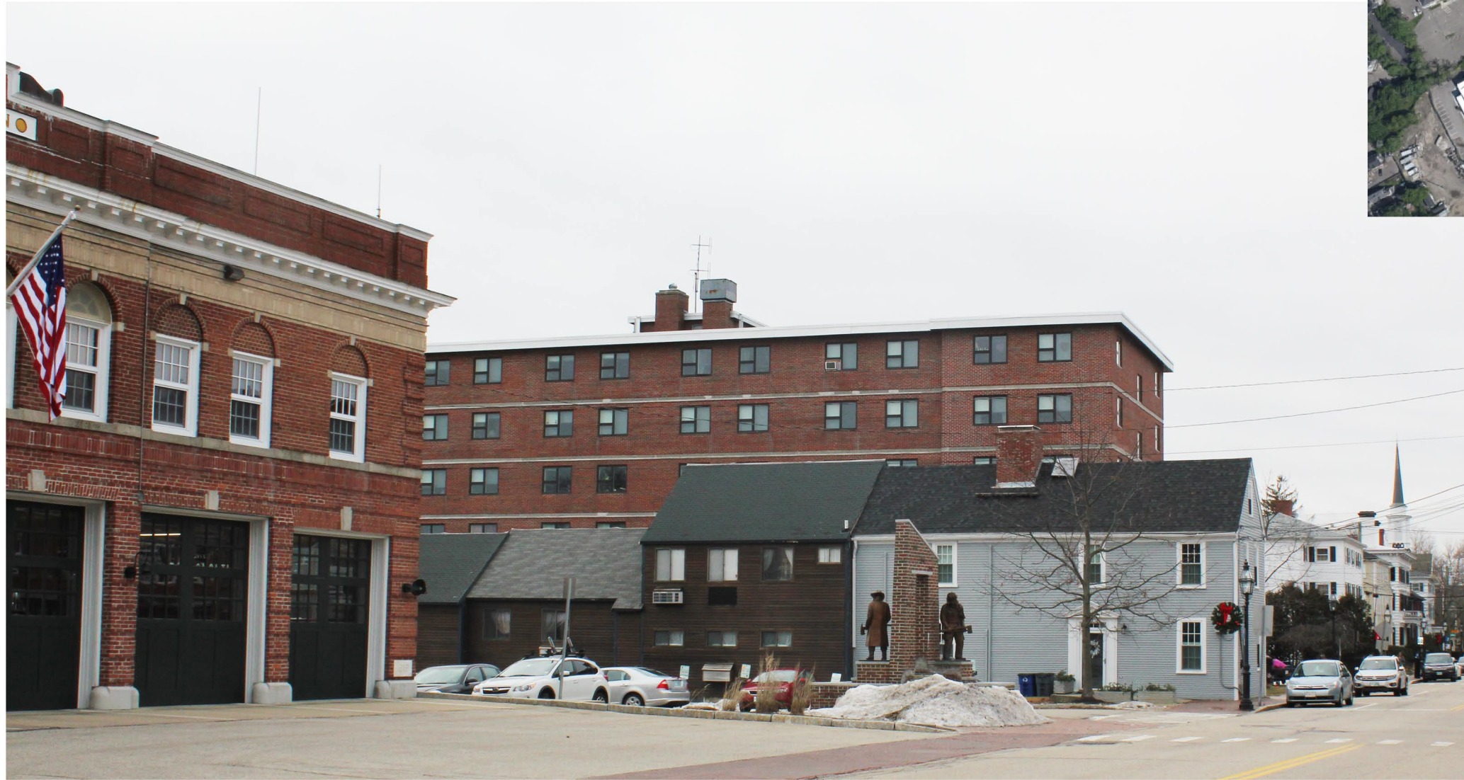
VIEW FROM COURT STREET
