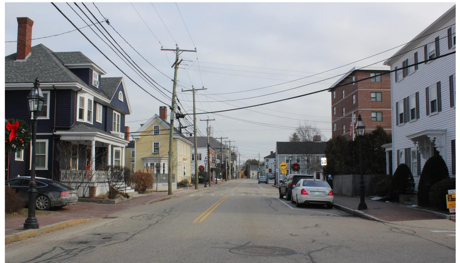
VIEW EAST DOWN COURT STREET
