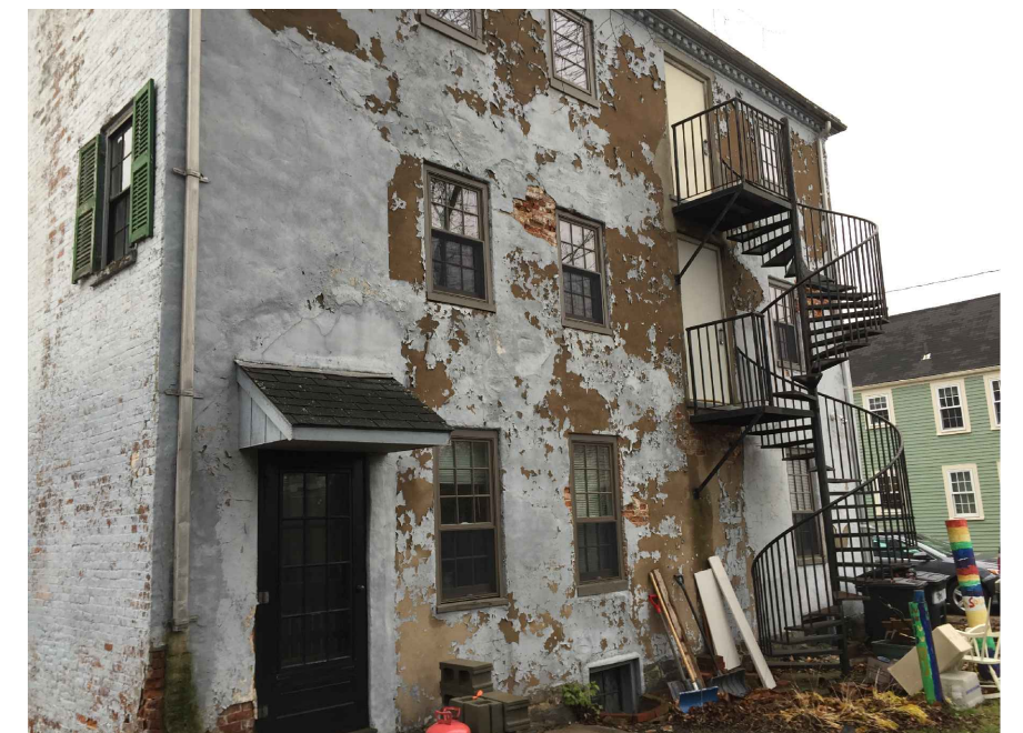
VIEW FROM REAR PROPERTY LINE
