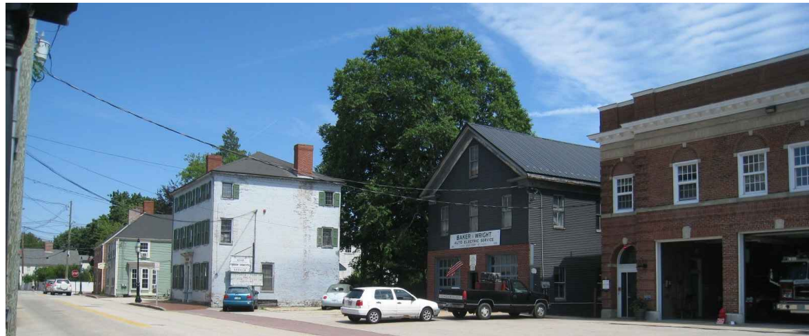
COURT STREET VIEW
