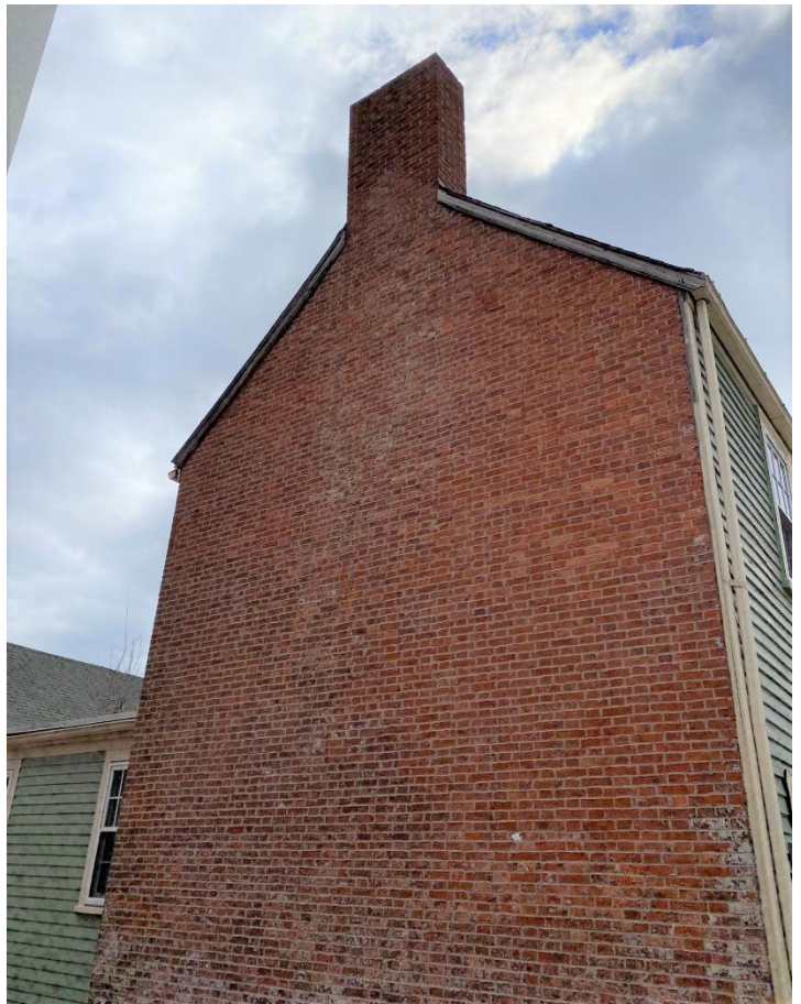
Figure 3. BHTNH HQ, East façade, showing full brick end wall and chimney of original section of building. The mural probably would be installed on the front lower quarter of the façade (lower right in this photo), but we do not yet have the artist's full proposal. Note evidence of surviving paint on the soft brick, suggesting that the wall was painted for at least a century after it was built, and possibly longer.
