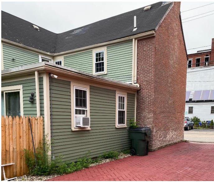
Figure 2. BHTNH HQ, East façade, showing brick end wall and one story addition.
