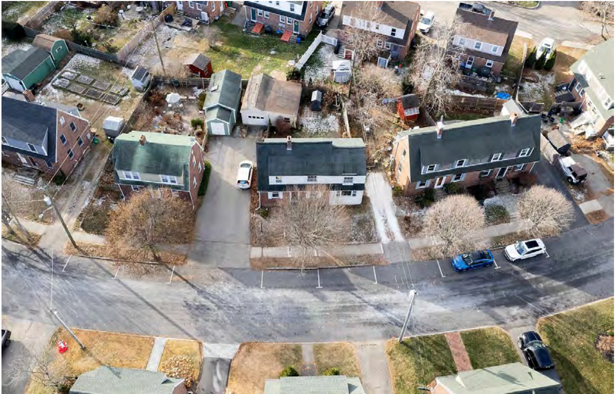
PHOTO 3: AERIAL VIEW OF PROPERTY. PROXIMITY VIEW. GARAGE ROOF AT END OF LIFE
