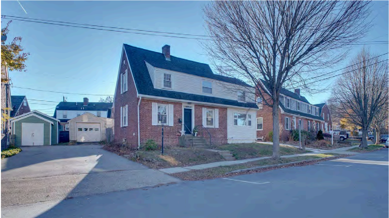
PHOTO 2: FRONT VIEW OF PROPERTY. GARAGE OPENING SHOWING VISIBLE SIGNS OF STRUCTURAL RACKING
