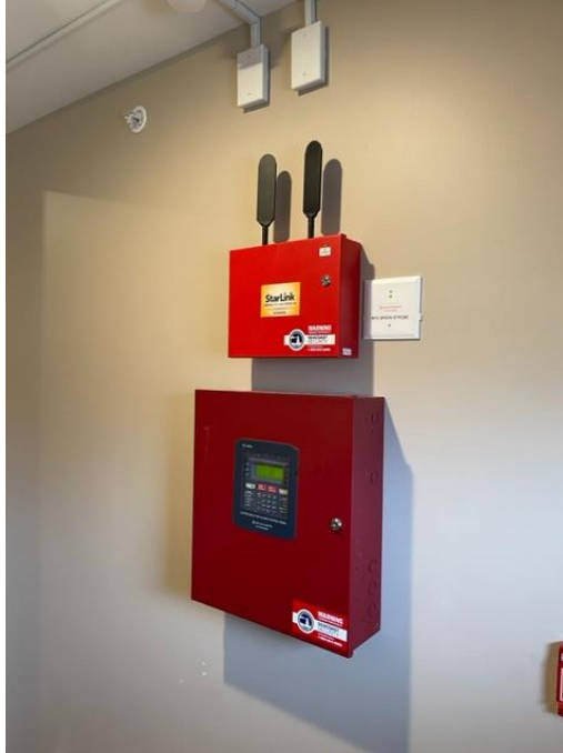
Figure 7. Fire Alarm Panel
