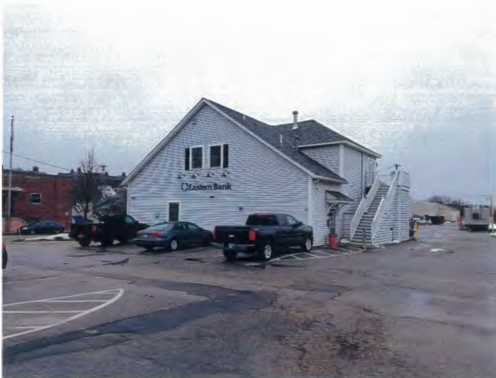
Existing Conditions - View of Property to the south (toward Bridge)
