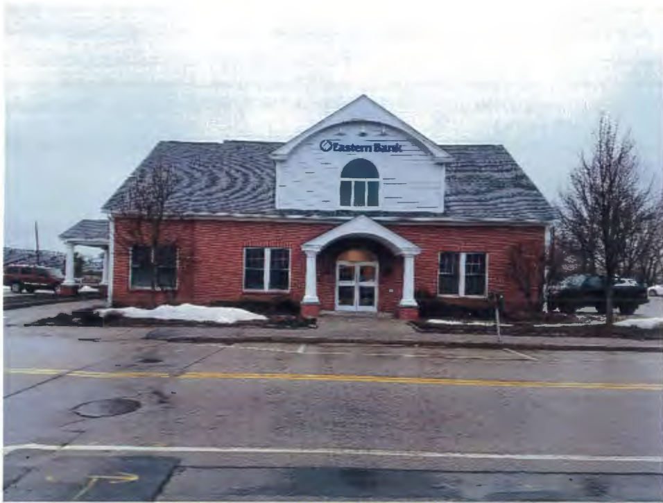
Existing Conditions - View of Property to the northwest (from Deer Street)
