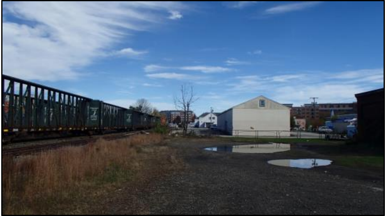
Plate 5. West Façade of Commercial Building, View East. The railroad tracks are to the north. This photograph was taken north of the structure in Plate 4 above. Note the brick building to the south.
