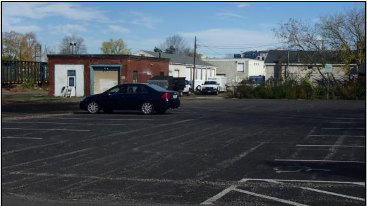
Plate 4. Brick Structure and Parking Lot with Railroad in Background, View North. This structure may be depicted on the 1850 map of Portsmouth as part of the railroad complex.
