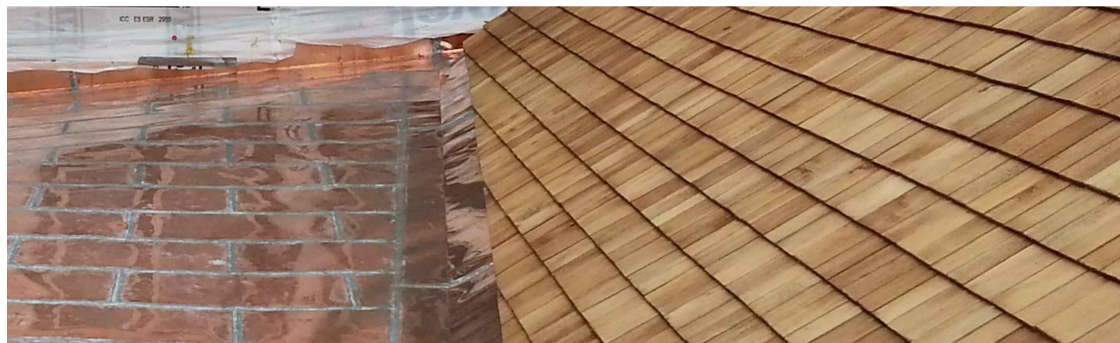
SOLDERED SEAM COPPER LOW SLOPE ROOF
