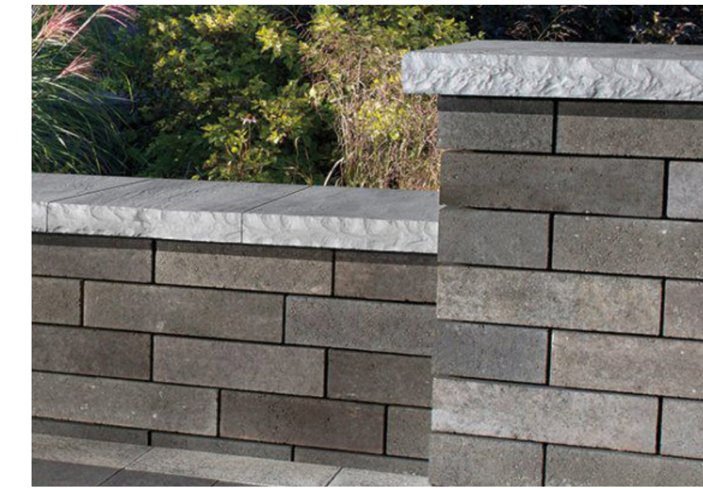
Cmu Seatwall With Granite Face And Cap
