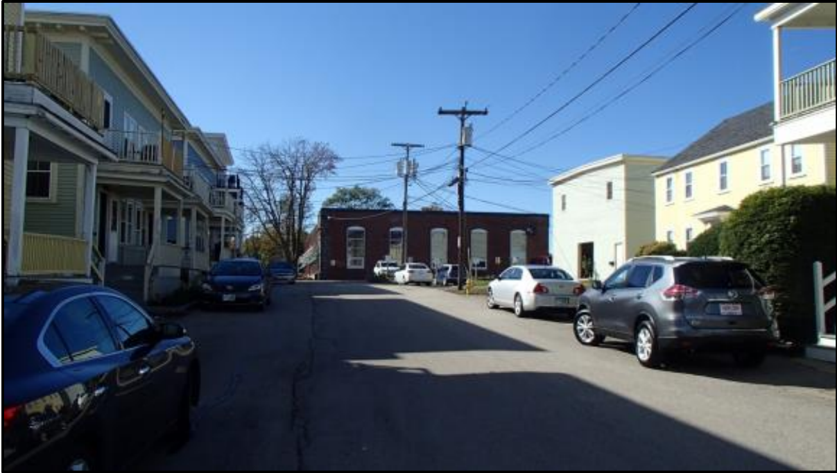
Plate 8. Hill Street, View West. The yellow dwelling and green garage on the north side of the street are in the project area. The brick building at the center of the picture, part of the Portsmouth Steam Factory, is not in the project area.
