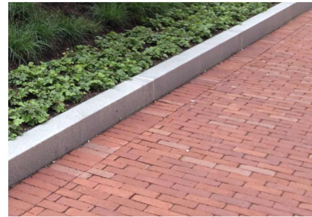
Brick Pavers With Granite Curb At Planter
