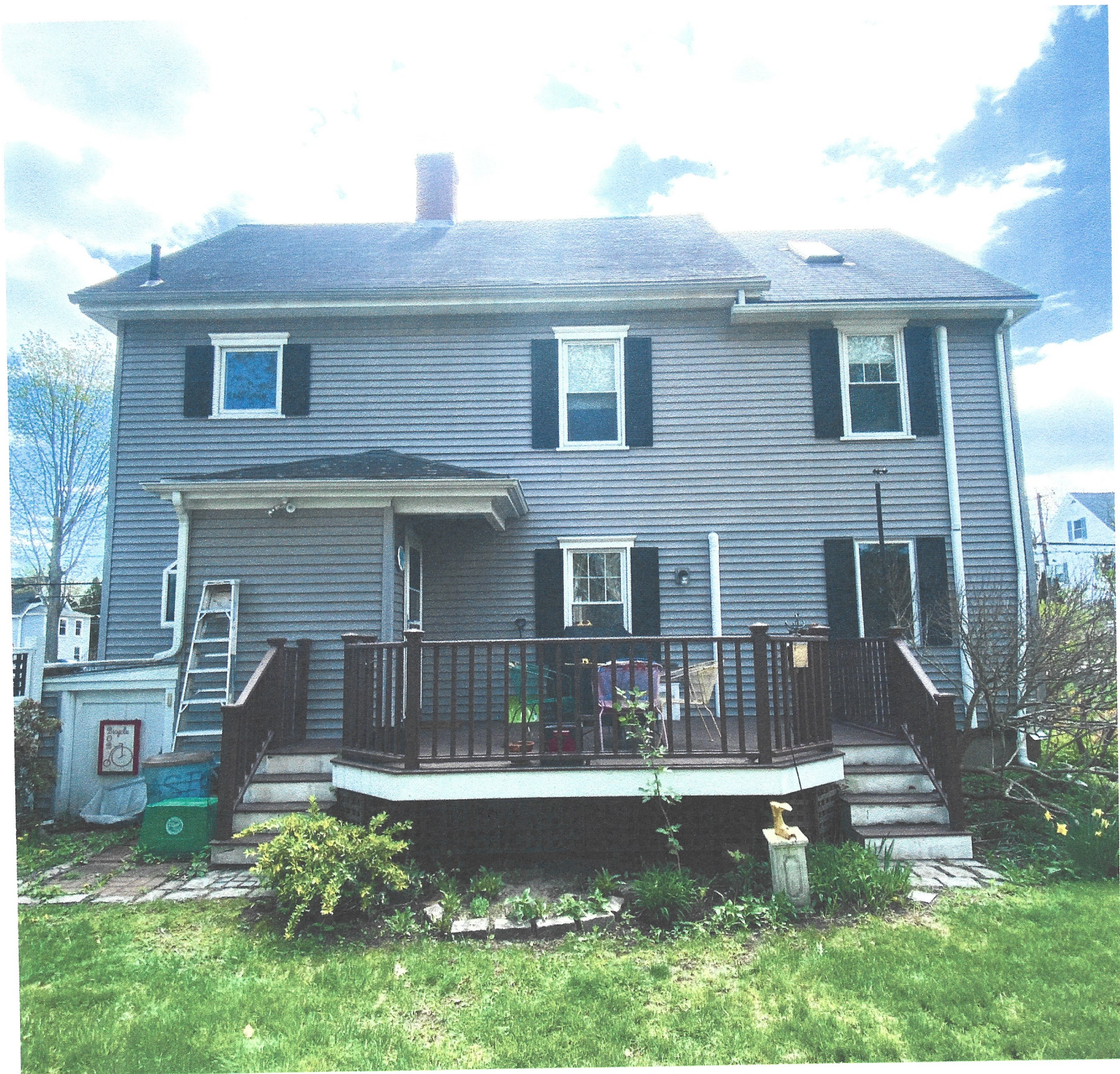
EXISTING REAR VIEW -1
