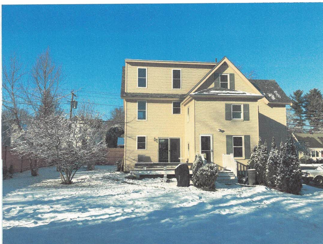
VIEW FROM RESIDENCE BACKYARD
