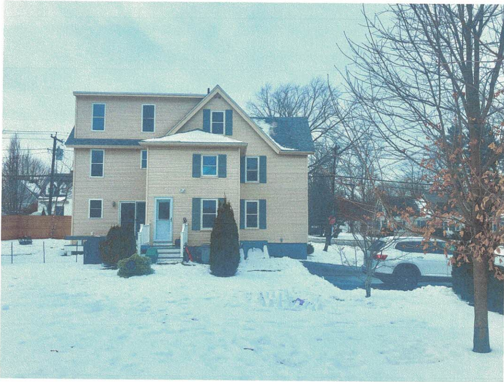
VIEW FROM RESIDENCE BACKYARD
