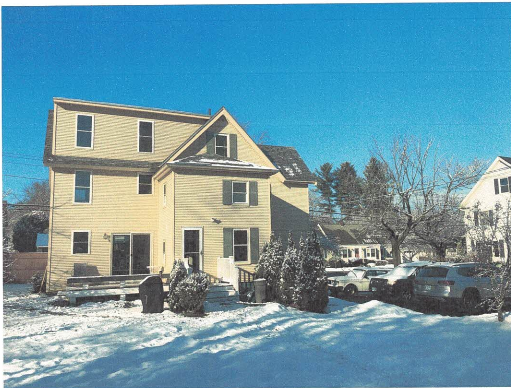
VIEW FROM RESIDENCE BACKYARD
