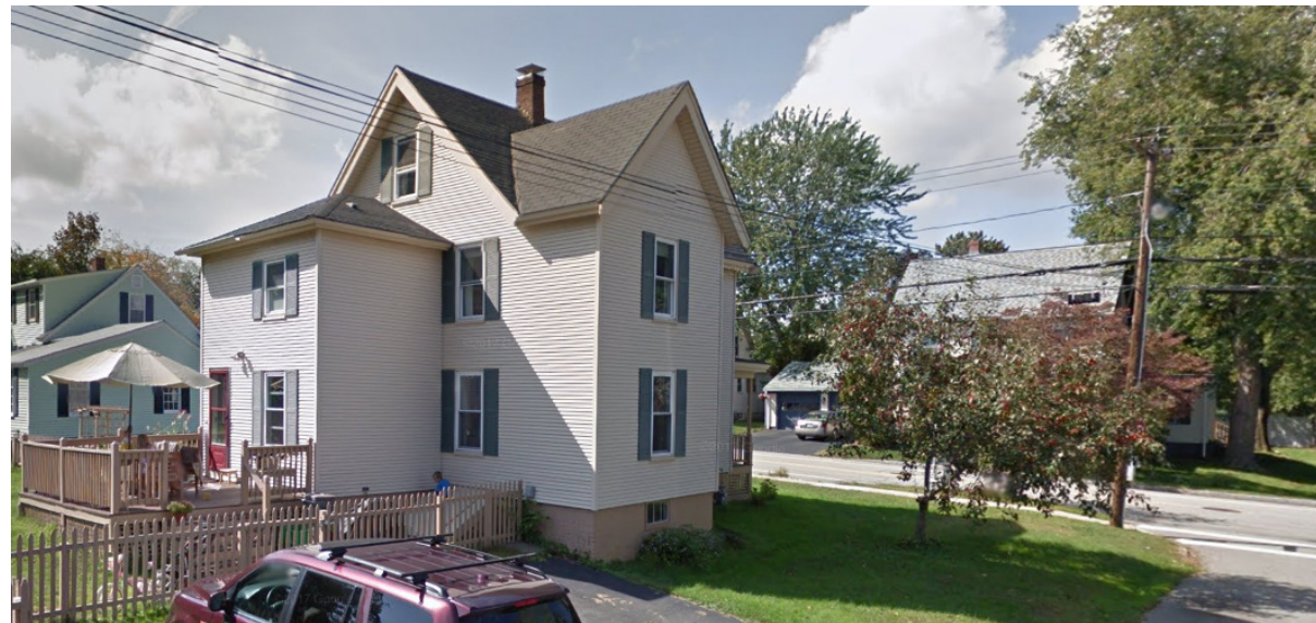
2) PHOTOGRAPH OF EXISTING STRUCTURE FROM WHIPPLE
