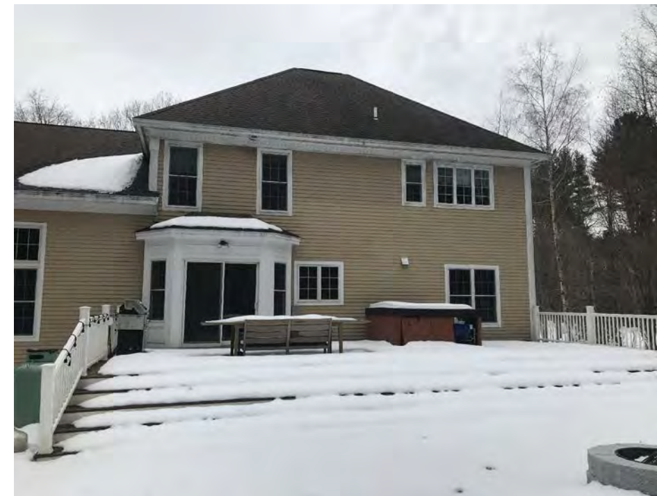
North/ Rear Deck Elevation
