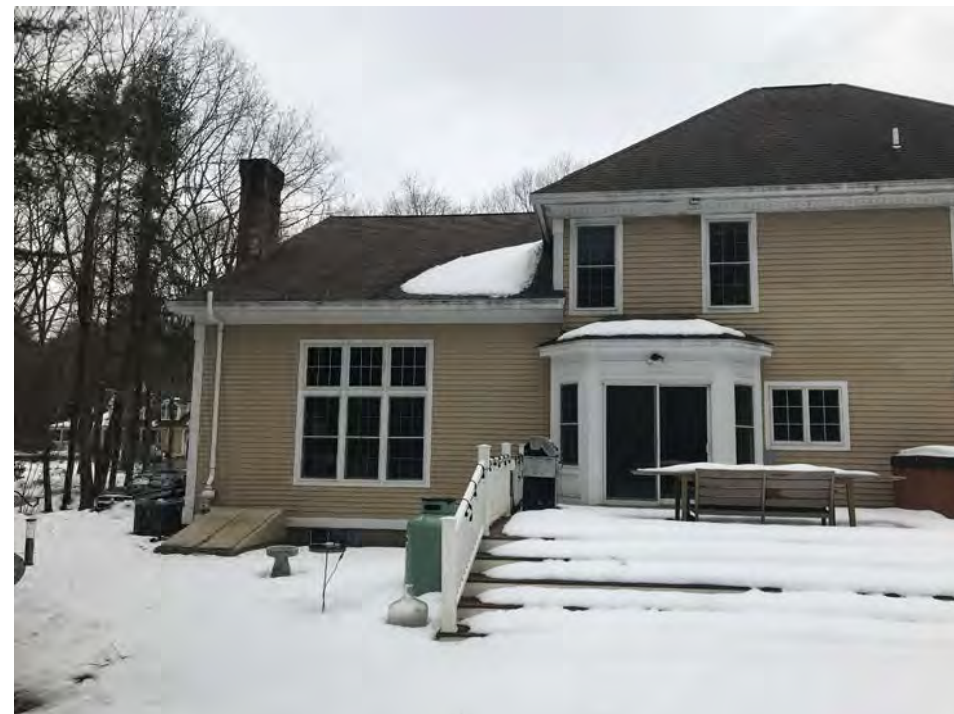
North/ Rear Deck Elevation
