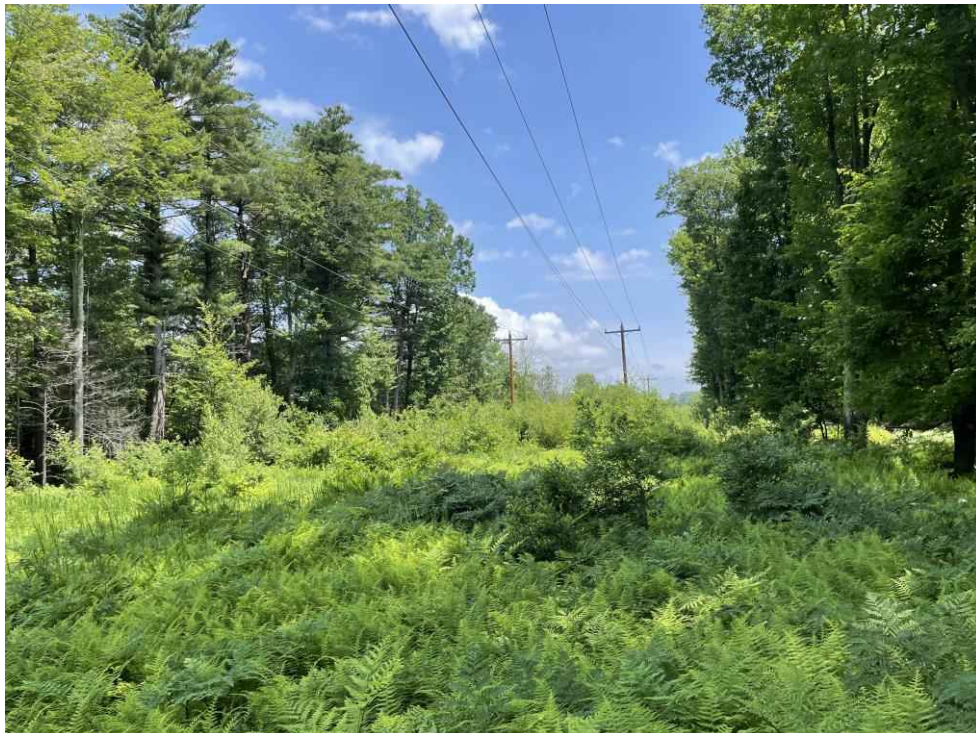
Photograph No. 10: Looking north towards Structure 86 on the 3171 Line ROW off Ocean Road, Portsmouth, NH.
