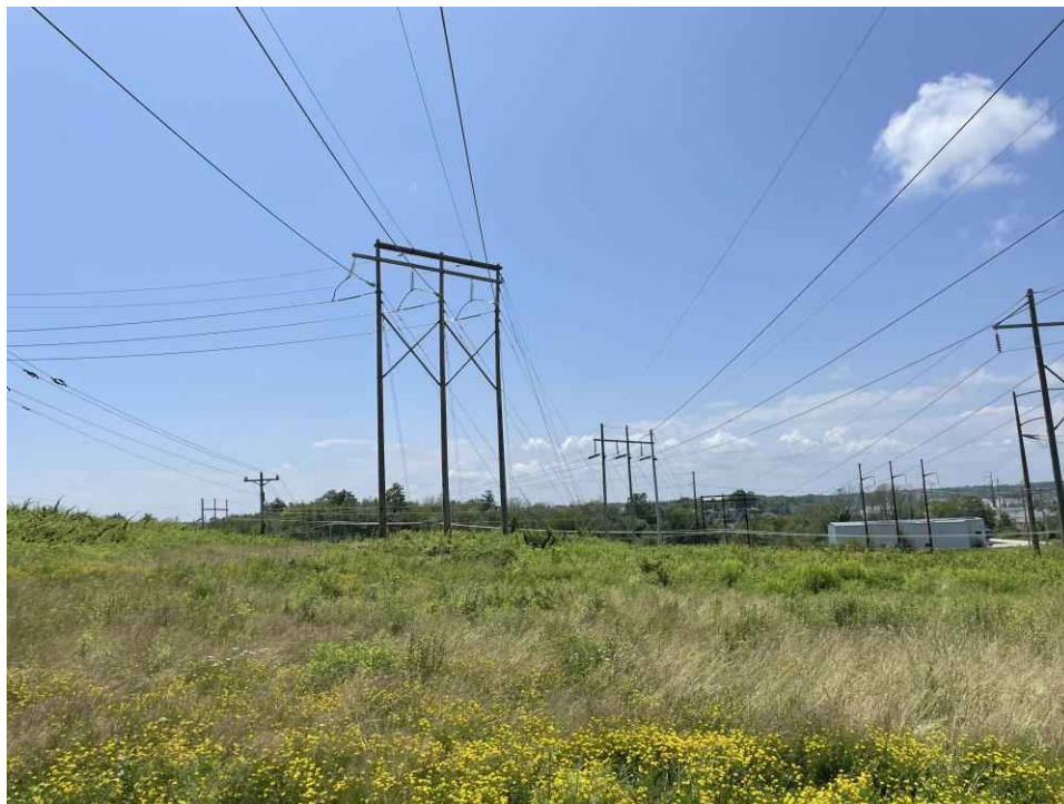
Photograph No. 24: Looking southwest at Structure 2 on the T13 Line ROW off Gosling Road, Portsmouth, NH.
