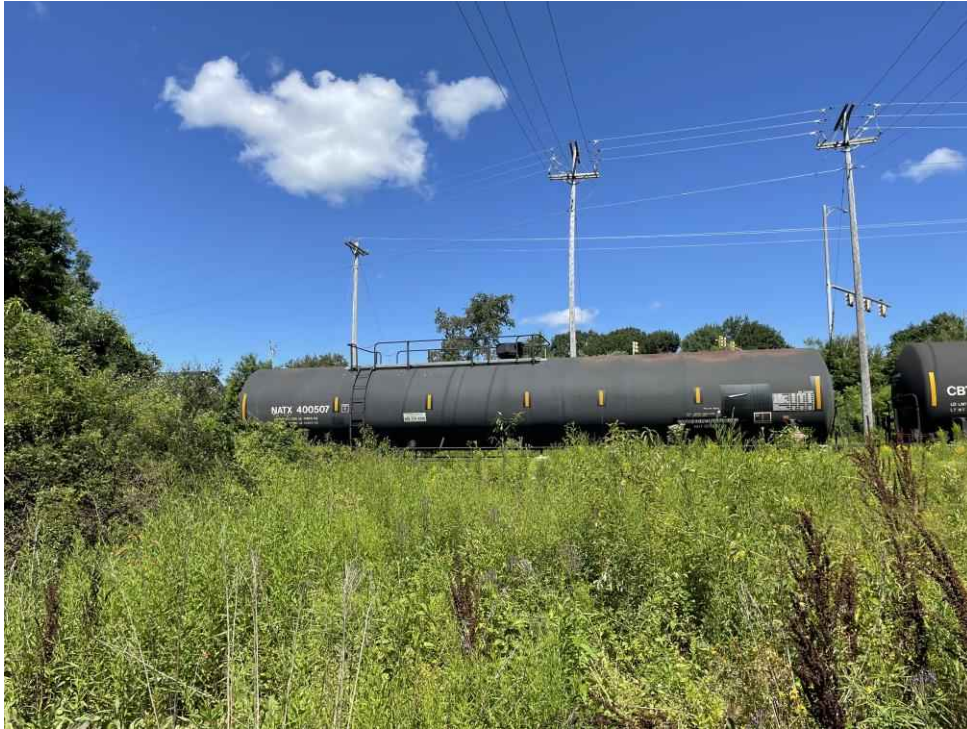
Photograph No. 19: Looking northwest towards Structures 72 and 72.6 on the 3171 Line ROW off NH33, Portsmouth, NH.
