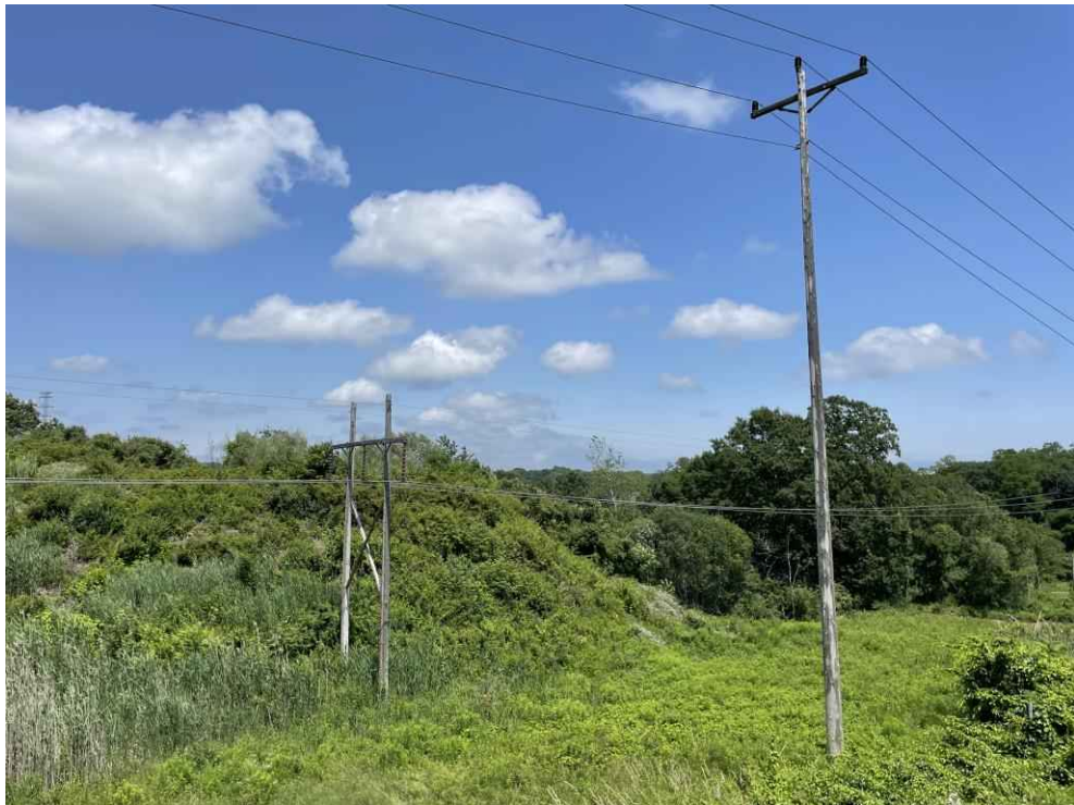
Photograph No. 34: Looking northeast at Structure 9 and Wetland PW-12 (PEM1/PSS1E) on the T13 Line ROW off Gosling Road, Portsmouth, NH.
