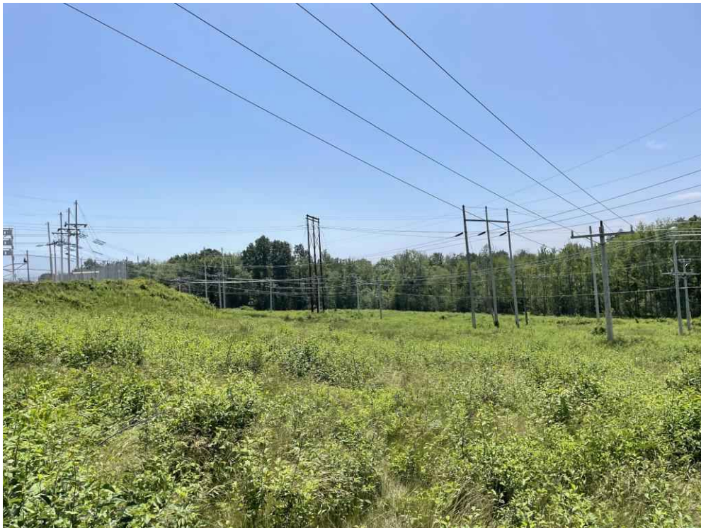
Photograph No. 26: Looking south at Structure 3 and Wetlands PW-5 (PEM1/PSS1E) and PW-6 (PEM1/PSS1E) on the T13 Line ROW off Gosling Road, Portsmouth, NH.
