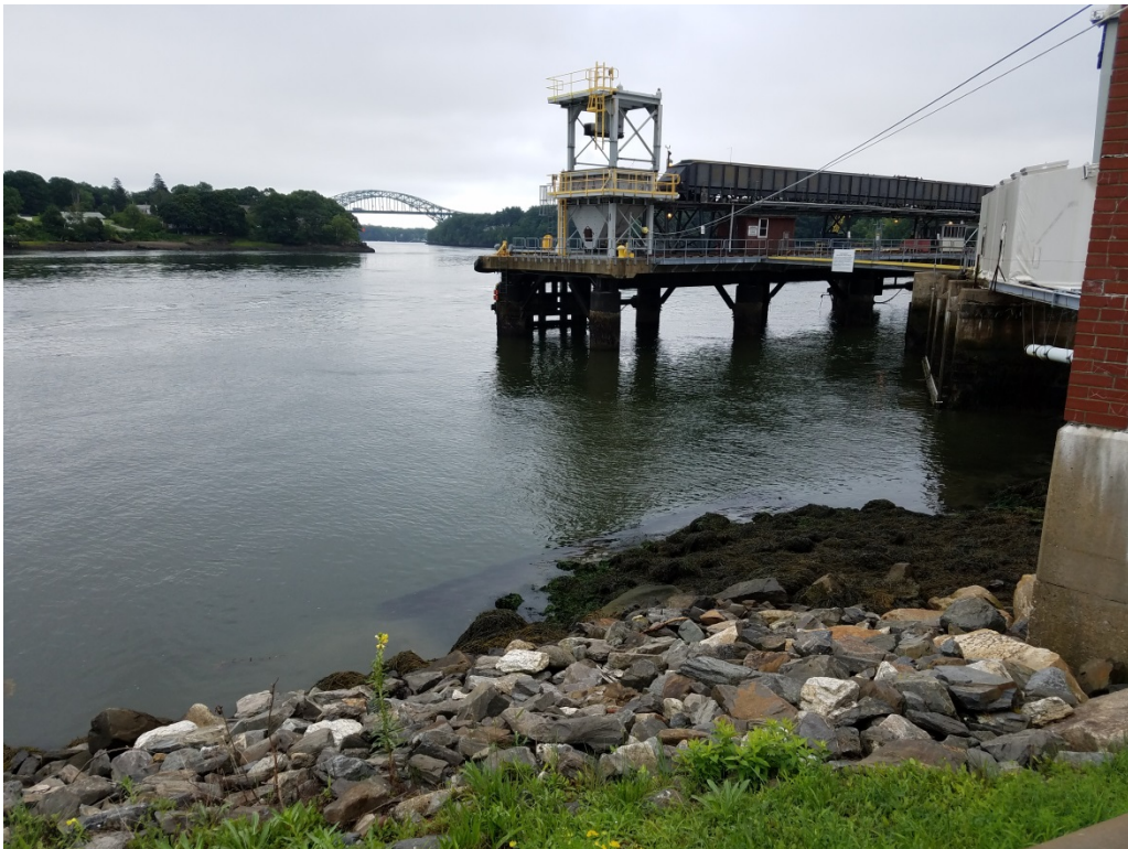
Photo 3. View of intakes 4, 5, and 6, facing southeast (intake hoses for test screens will enter at unit 4)
