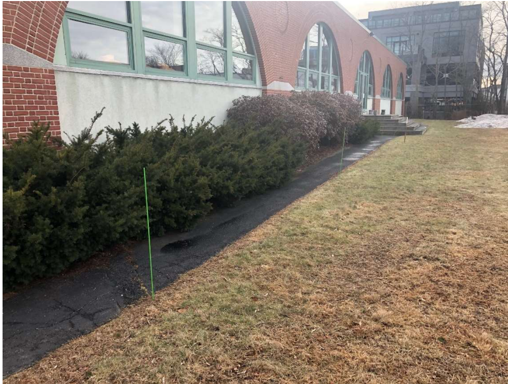
Photo #3: Looking southwest along existing building within 100-foot tidal wetland buffer.
