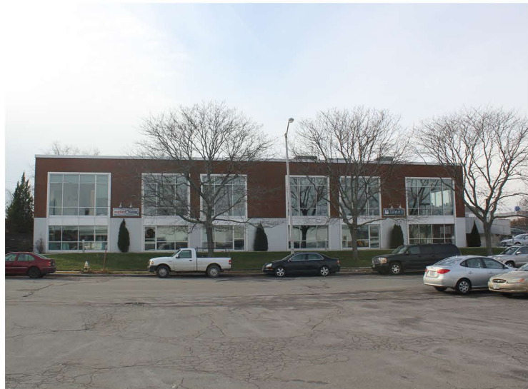
15 EXISTING 111 MAPLEWOOD AVENUE
