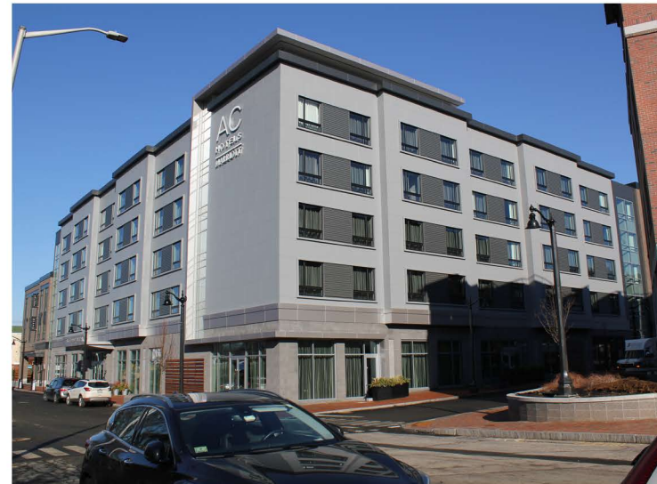
21 EXISTING 299 VAUGHAN STREET
