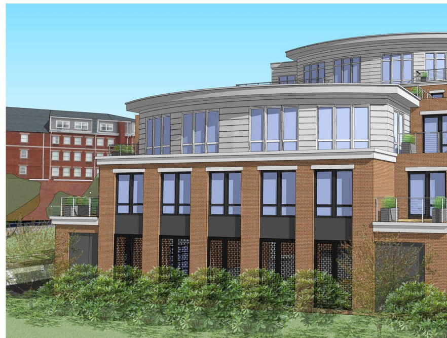
THE CURVED NAUTICAL THEME CONTINUES TO STEP TOWARD NORTH MILL POND AND IS SET BACK FROM THE MASONRY PILARS BELOW. THE BRICK OPENINGS HAVE BEEN CAPPED WITH PRECAST LINTELS TO ADD DETAIL AND DIMENSION.
