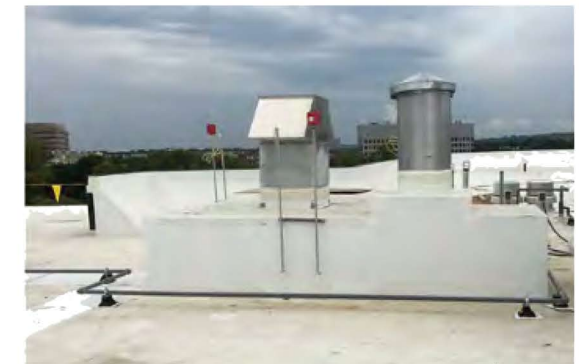
ELEVATOR OVERRUN AND VENT
