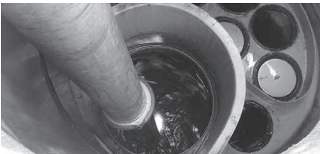
Vacuuming Sump Through MAW
