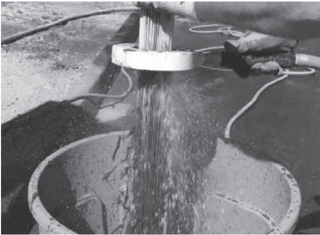
Rinsing Cartridge with Contech Rinse Tool
