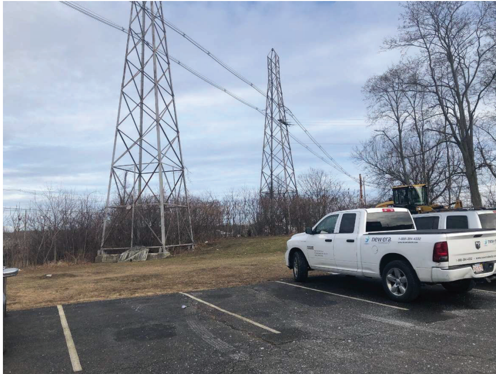
Photo #1: Looking northeast at existing utility towers and parking located in 100-foot tidal wetland buffer.
