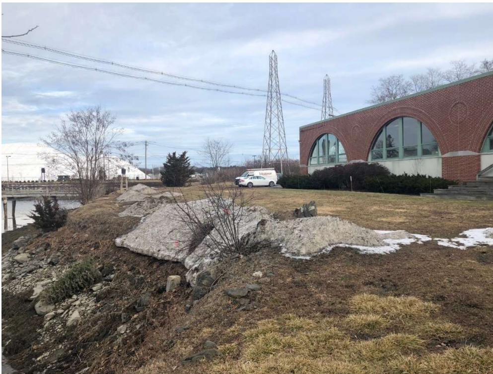
Photo #4: Looking northeast toward existing building and parking located in 100-foot tidal wetland buffer.
