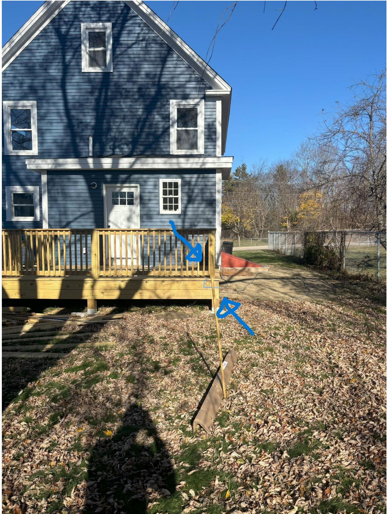
Rear Yard View of Deck
