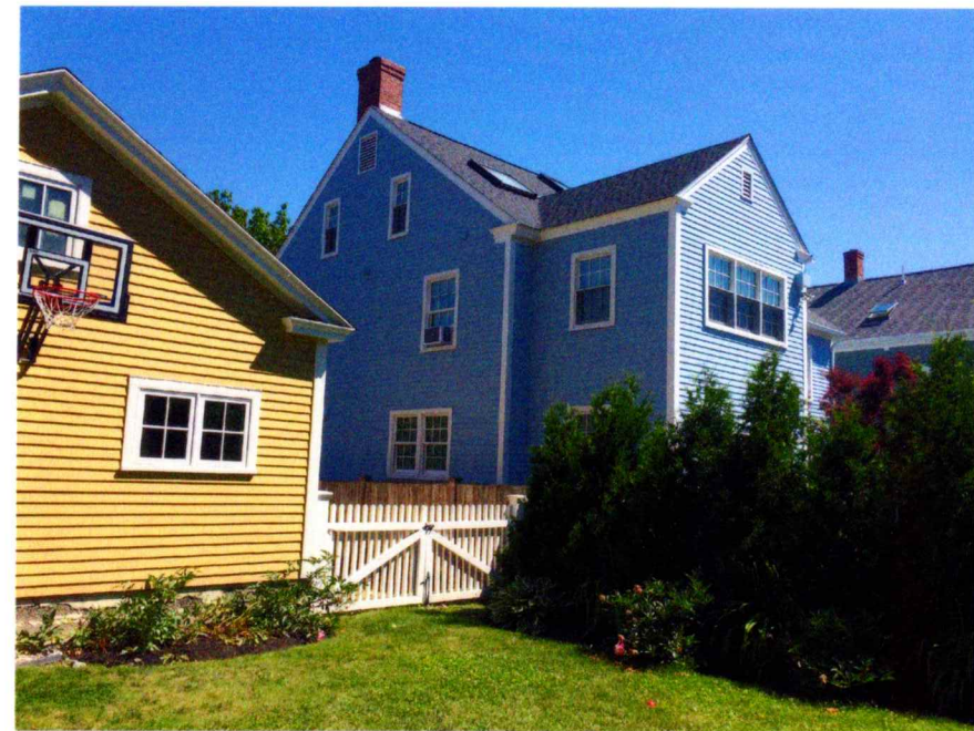
2 VIEWS OF REAR ELEVATION
