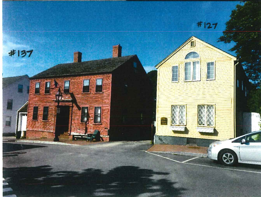
VIEW FROM HIGH STREET
