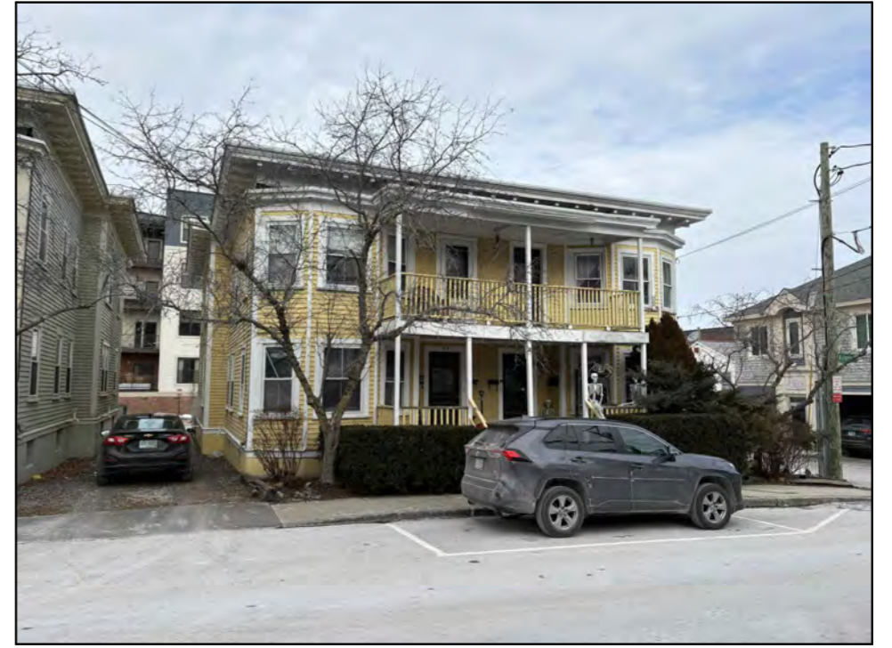
HANOVER STREET ELEVATION OF 319 HANOVER STREET
