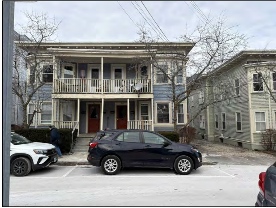
HANOVER STREET ELEVATION OF 339 HANOVER STREET
