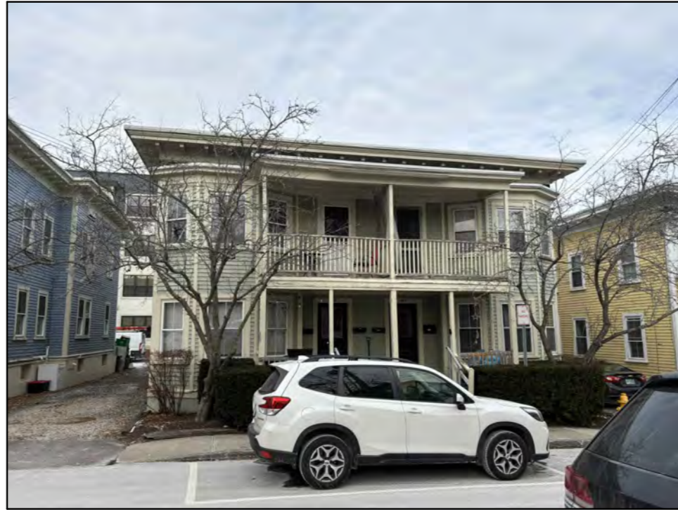
HANOVER STREET ELEVATION OF 329 HANOVER STREET
