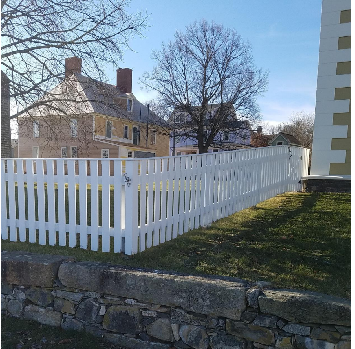
Wentworth-Gardner House Existing Fencing (view from Mechanic Street)
