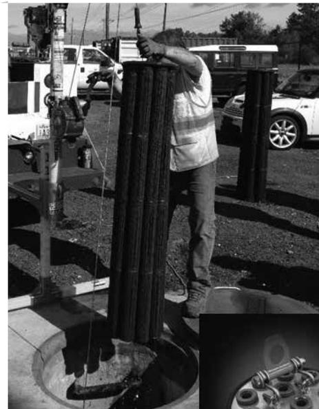
Cartridge Removal & Lifting Device
