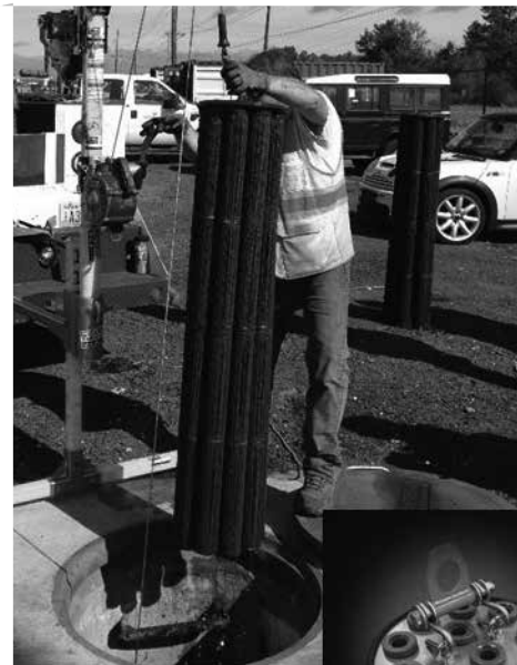
Cartridge Removal & Lifting Device
