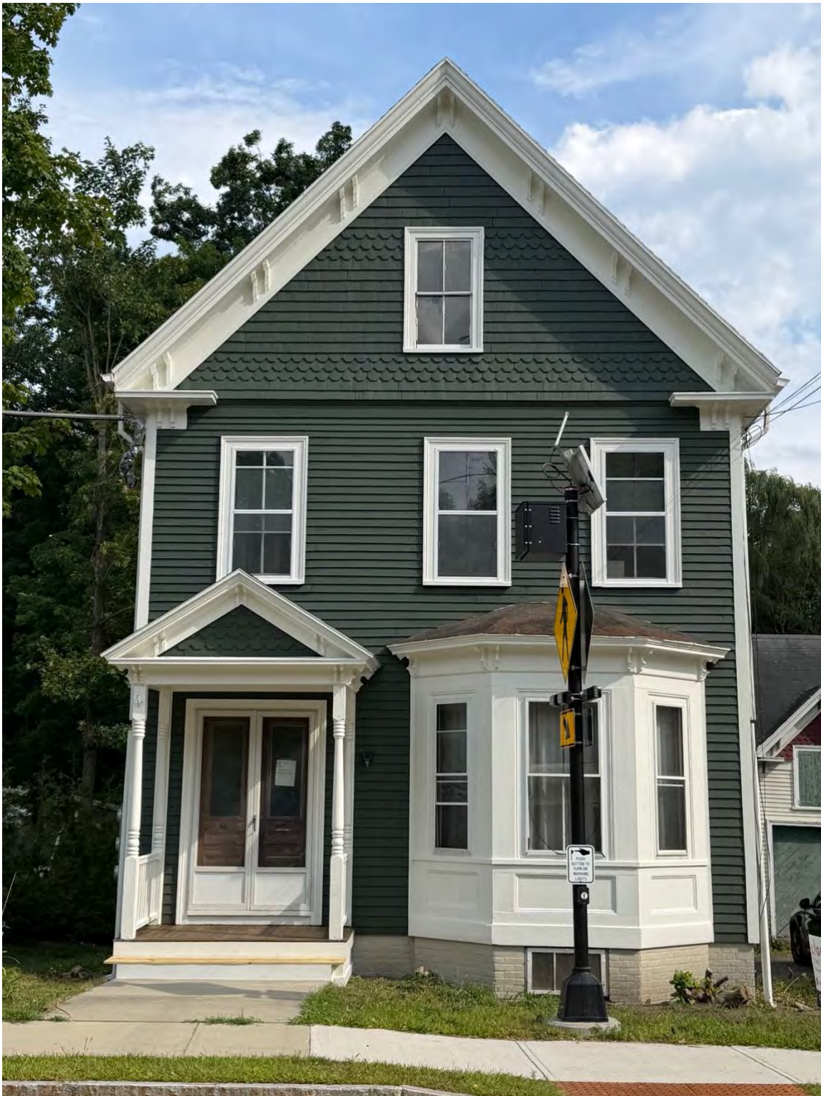
Current Photos Front of House with City-Installed Crossing Sign
