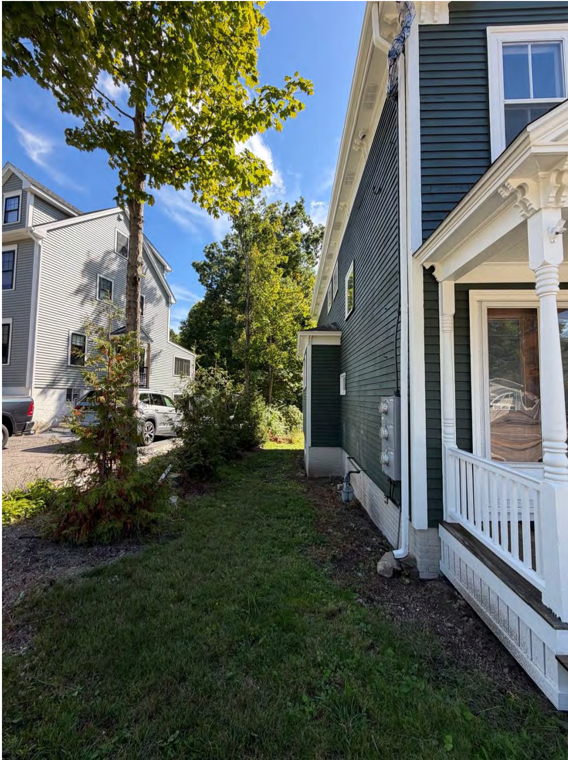
Left (North) Boundary of Property View from Islington Street
