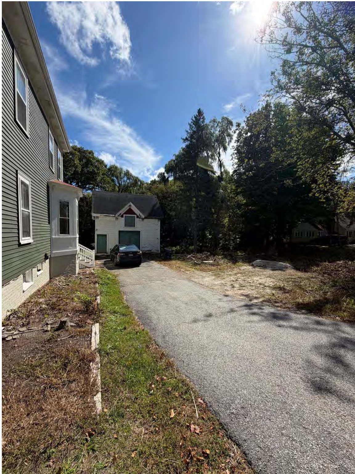
Right (South) Side of House - Driveway with 6 Parking Spaces
