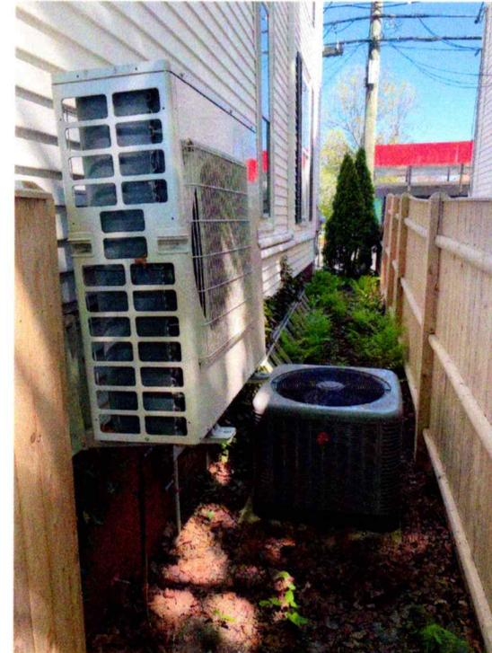
Lower Exist Heat Pump & Add single Heat Pump, relocated from Right Side. The 2 Exist Units on the Right Side will be replaced with 1 Unit. Both will be ground mounted. Exist AC Condenser to remain.
