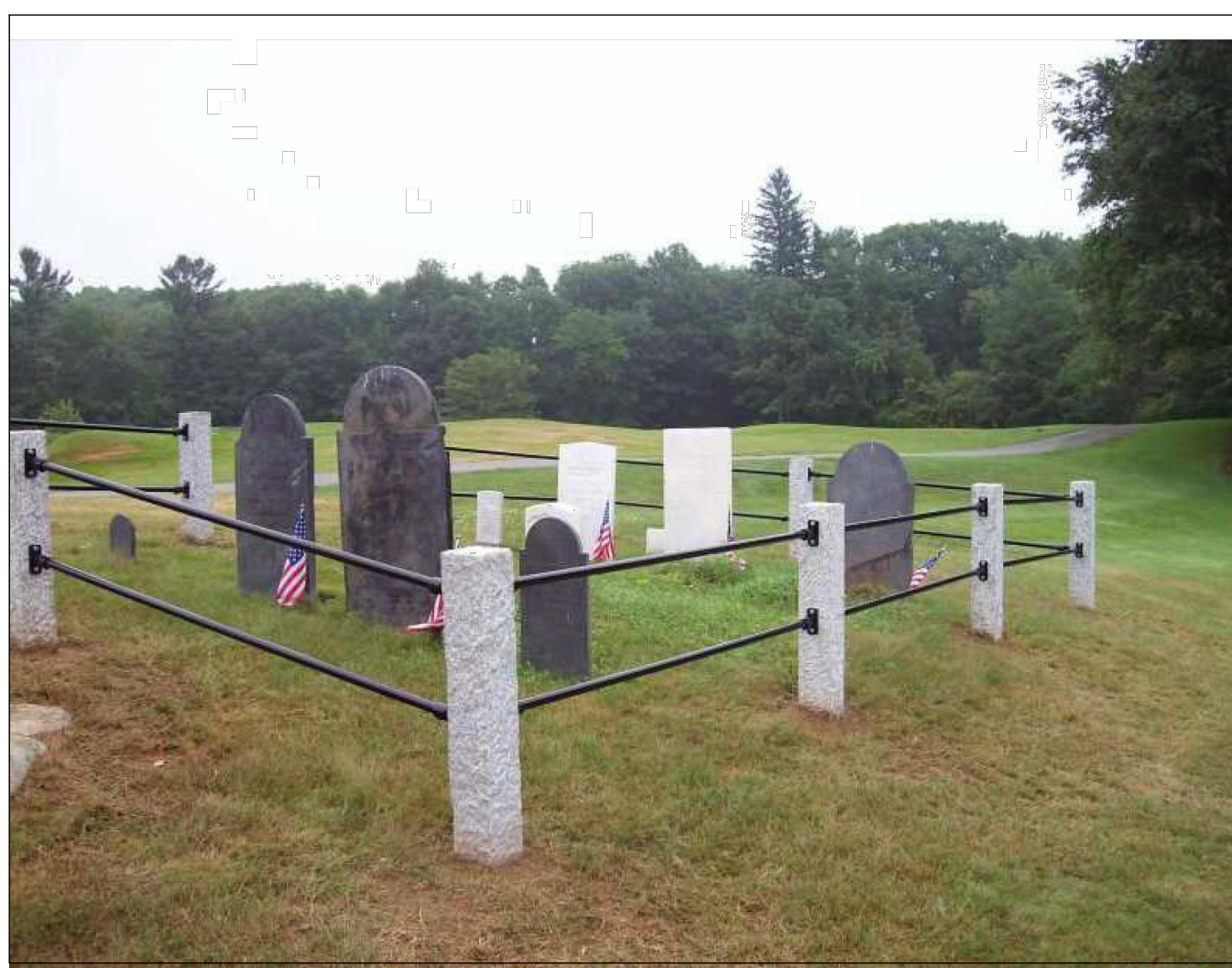
Proposed Memorial and Cemetery Fence - 8x8 granite posts with 2.5" diameter metal rails.
