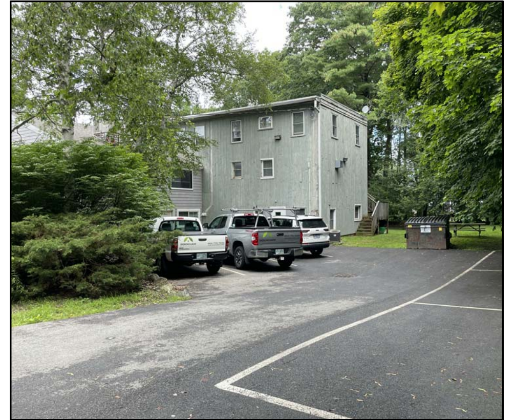
2059 LAFAYETTE ROAD LOOKING NORTH
