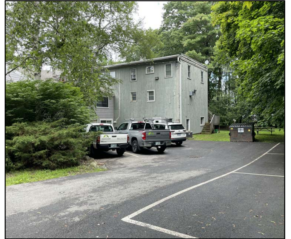
2059 LAFAYETTE ROAD LOOKING NORTH
