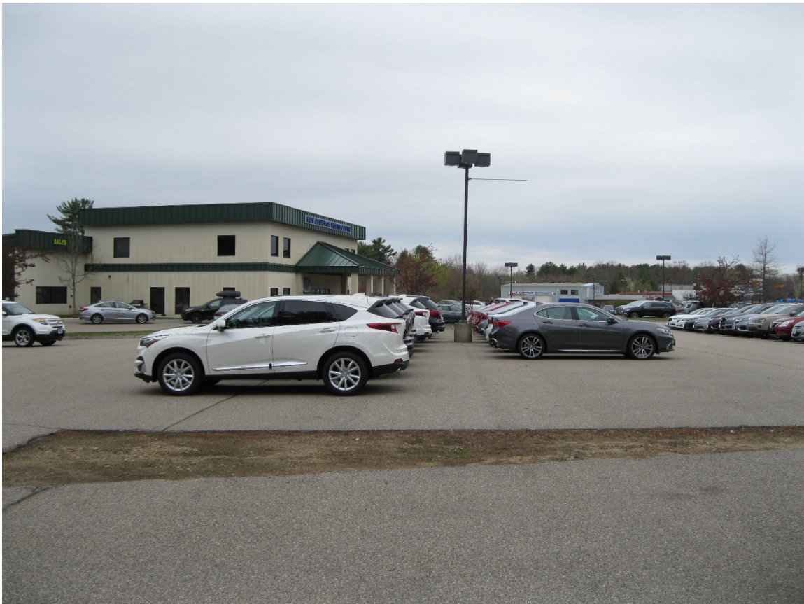
Facing the easterly side of building from parking lot
