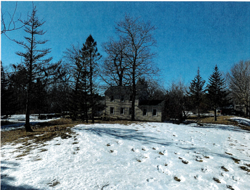
Existing Conditions – View of Property from the South
