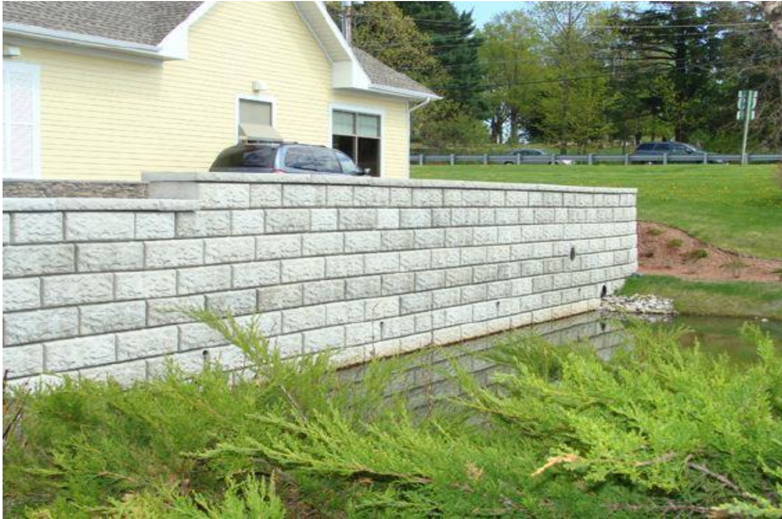
Rear Retaining Wall: Genest London Boulder Retaining Wall Blocks and Caps
